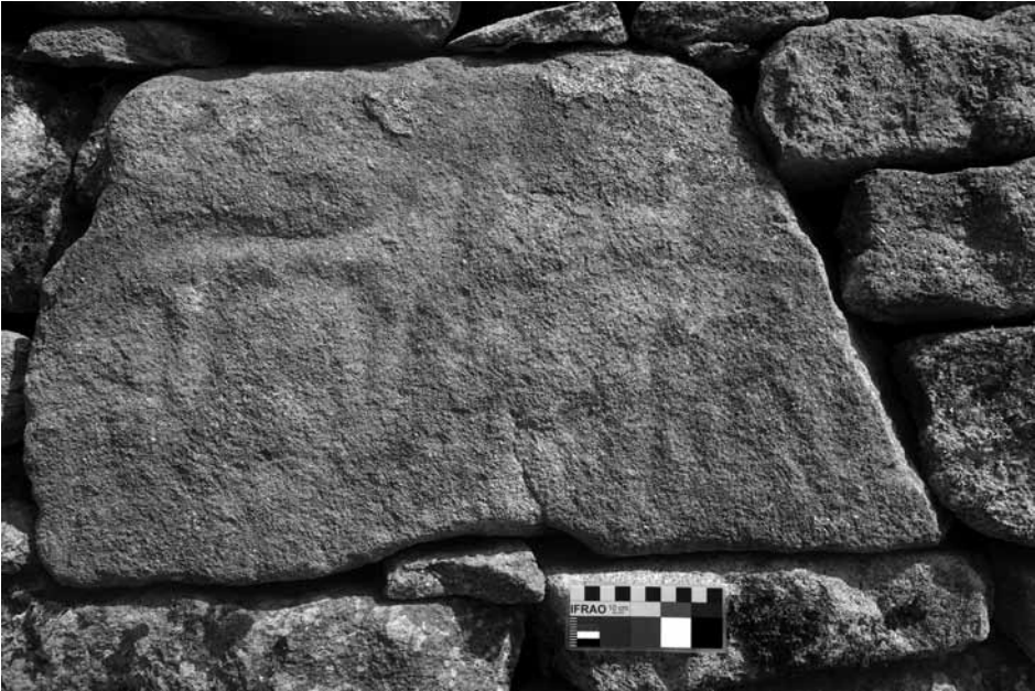
Fig. 2 – Zoomorphs on the Castro walls, showing the amount of weathering experienced by granite in one or two millennia
